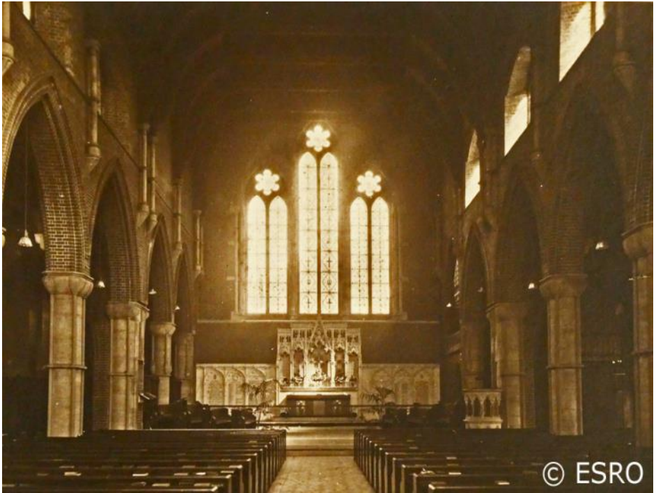
Photograph taken in 1922 showing the interior of St Matthew's Church with the newly installed reredos brought from St Peter's Church
