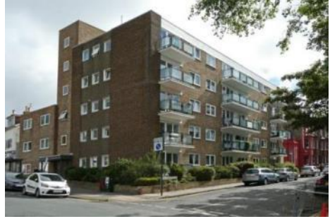
St. Matthew's Court Flats on the site of St. Matthew's Church
