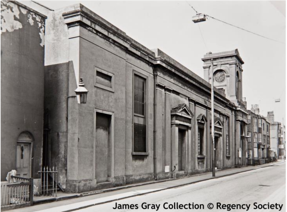
All Souls' Church in 1967 shortly before its demolition
