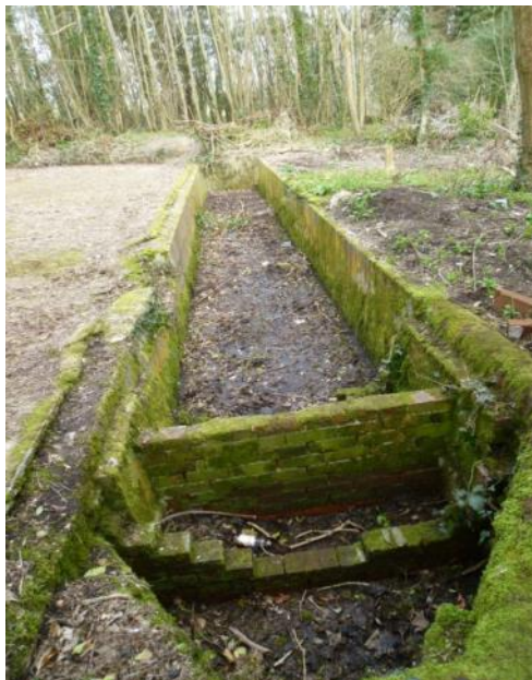
Rainwater Collecting Channel © 2015
