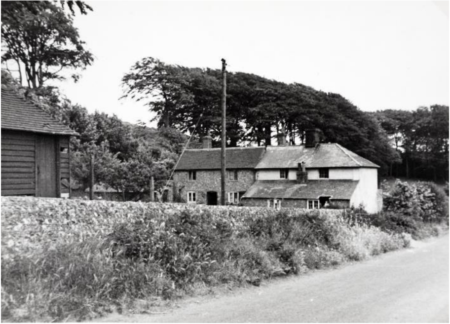
The Menagerie Farm Cottages on the east side of Coldean Lane from the James Gray Collection © The Regency Society
