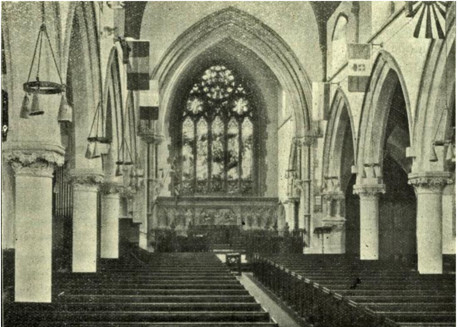
A photograph of the church c1915 showing the columns and arches which supported the roof.
